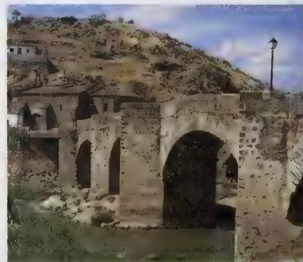
Bridge of San Lázaro over the Jerte River at Plasencia, Spain
